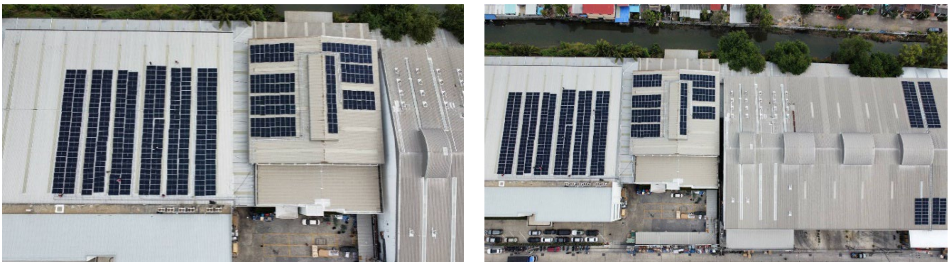
(Installation of solar rooftop power generation systems)
